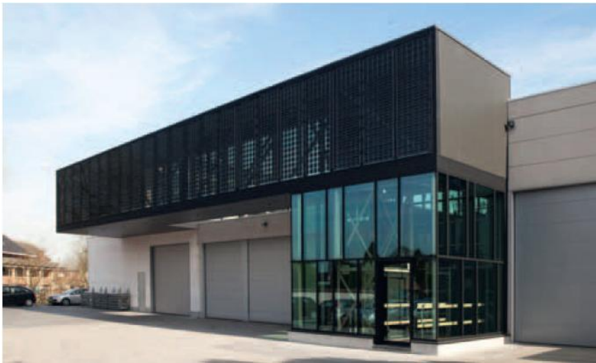
Figure 3.4.2.1: BIPV façade of Vandepuut office in Oosterzele, Belgium. (SAPA Building System 2012)
