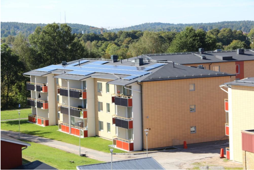
Figure 3.7.1.4: The final result of the renovation of Brogården. (Skanska 2014)
