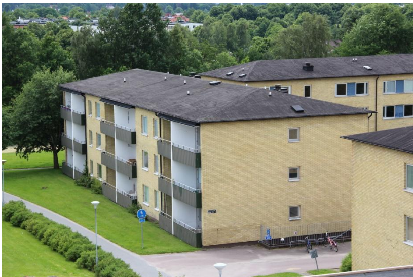
Figure 3.7.1.1: Before the renovation with ELEMENTUM eco elements (Skanska 2014).
