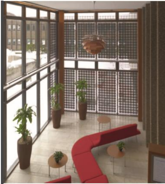
Figure 3.4.1.1: Integrated SAPA Solar BIPV in the façade of head entrance of Partille Municipal Office in Sweden. (SAPA Building System 2012)
