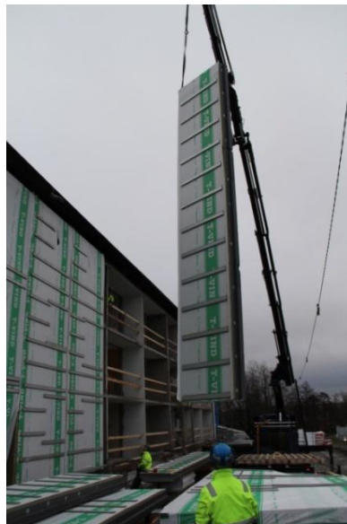
Figure 3.7.1.3: Mounting of the prefabricated ELEMENTUM façade elements at Brogårdén, stage three (Skanska 2014).
