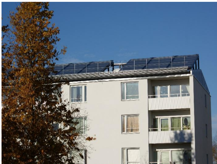
Figure 3.3.1.3: The final result after renovating with Smartfront (Smartfront 2015).
