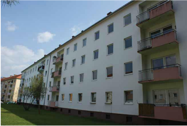
Figure 3.1.3.1: Kapfenberg building before renovation. (AEE INTEC 2015)
