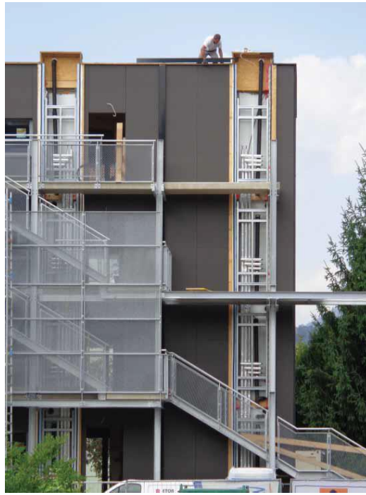
Figure 3.1.3.2: Picture of the integrated elements with building services, without the external layer (AEE INTEC 2015).
