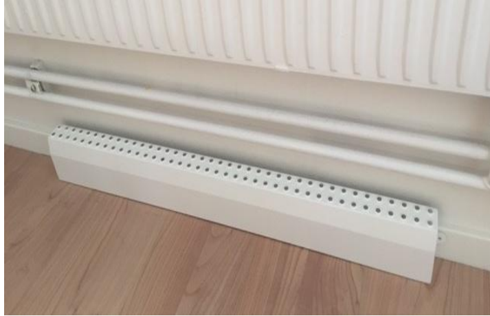
Figure 3.3.2: Smartfront's supply air device (Smartfront 2016).
