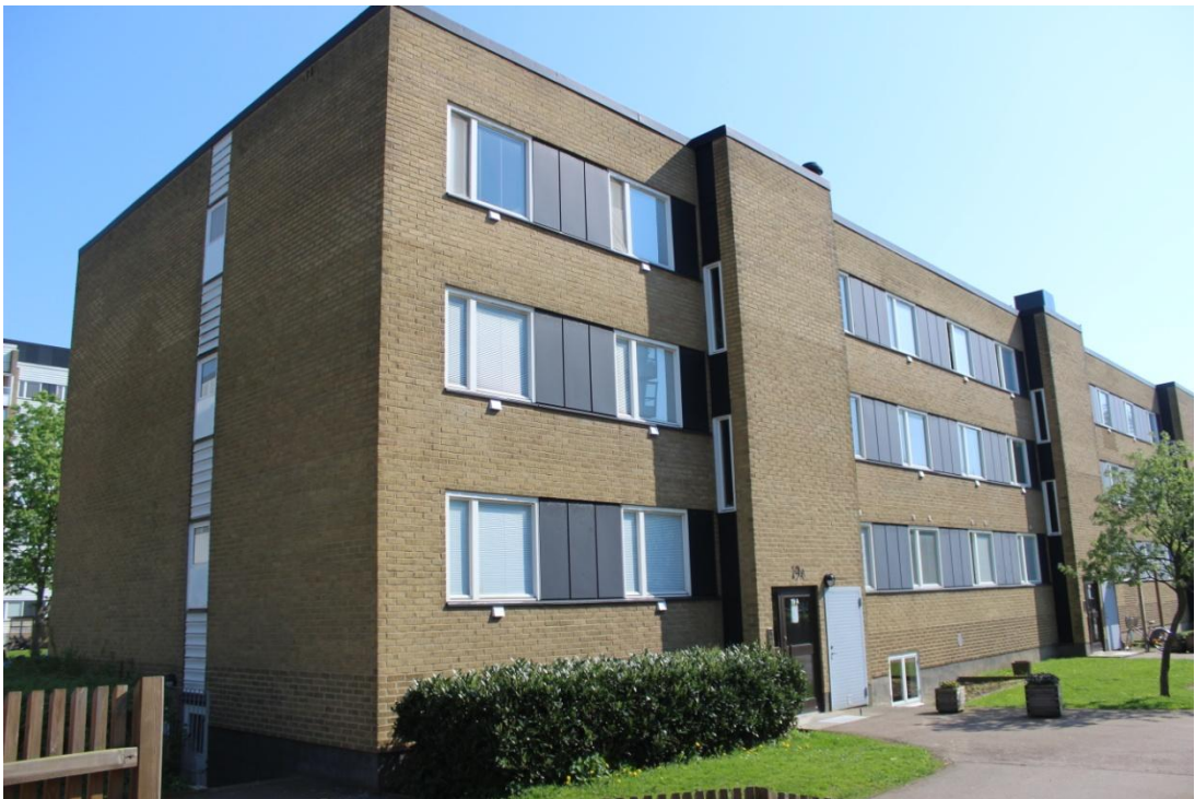
Figure 4.1.4: The end wall and northwest oriented façade of the reference house.
