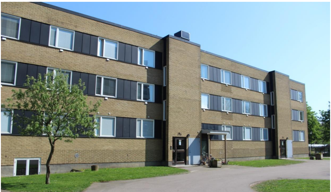
Figure 4.1.3: The northwest oriented façade of the reference house.
