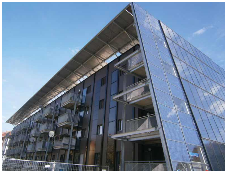
Figure 3.1.3.3: Kapfenberg after renovation, notice the integration of the covering of the building service elements (AEE INTEC 2015).
