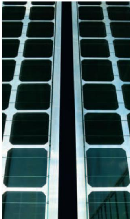
Figure 3.4.2.2: BIPV façade elements (SAPA Building System 2012).
