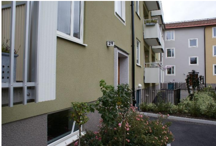
Figure 3.3.2.1: The façade of the buildings in the neighbourhood of Landsfogden after the renovation using Smartfront. (Smartfront 2016)
