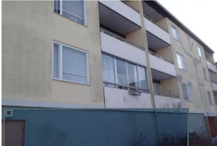
Figure 3.3.1.1: Lagersberg before the renovation (Smartfront 2015).
