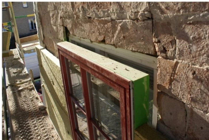
Figure 3.3.3: Window mounted outside the existing window using mounting frames (Smartfront 2016).
