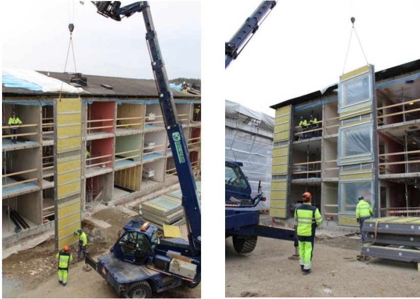
Figure 3.7.1.2: Mounting of the built on site ELEMENTUM façade elements at Brogårdén, stage one (Skanska 2014).
